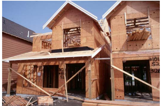
Figure 1 - Light wood-framing construction site
