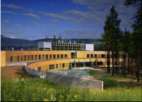
Nicola Valley Institute of Technology Phase I, Merritt, BC Busby + Associates Architects
